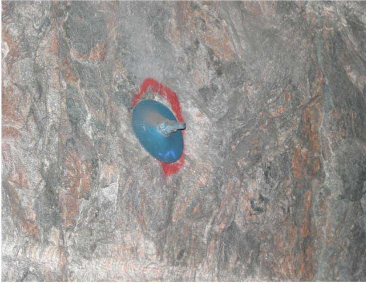
Figure 6-3. A reinforcement bolt with a protective coating of powder paint and epoxy in the Frøya Tunnel in Norway (Photo: Fredrik Mossmark).
