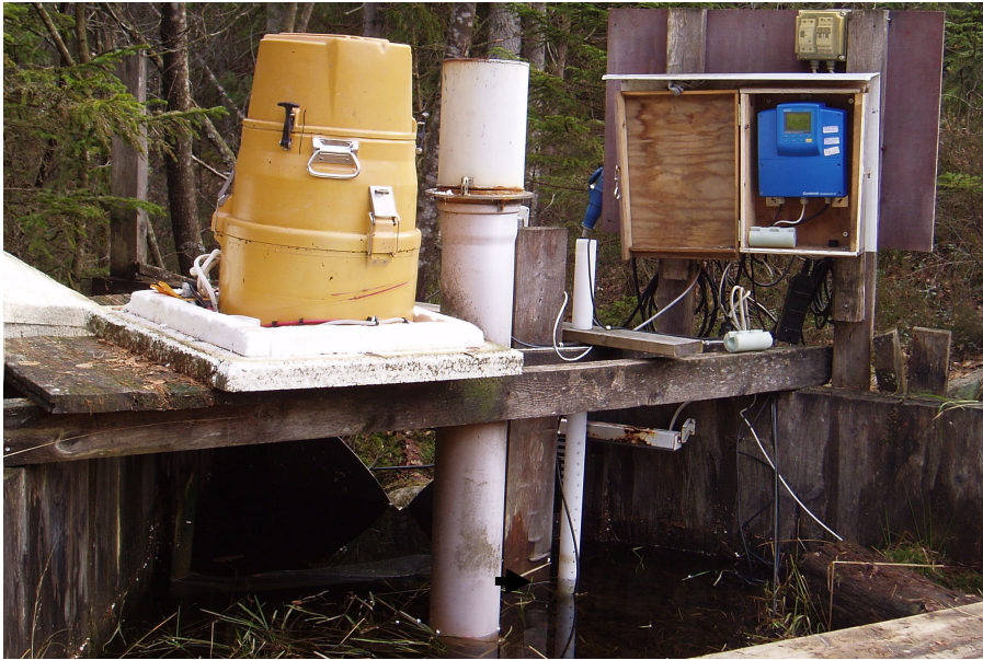
Figure 7-1. V-notched weir with water level recorder at the F3 catchment. An automatic water sampler (on top) and a pH and EC logger are installed at this weir.
